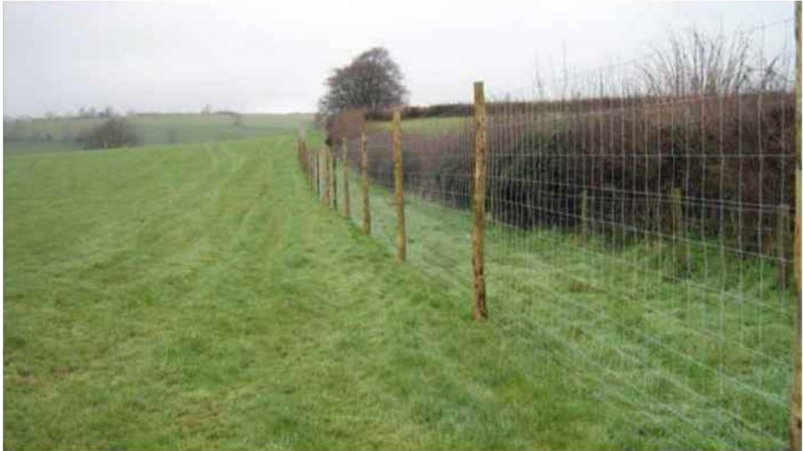
Figure 4.5: Typical Deer Fencing
